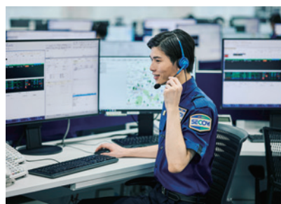
SECOM control center
