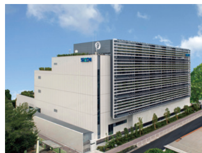
Exterior of the TC4 Secure Data Center®
