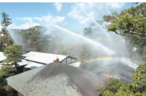
Water cannon test (Nohmi Bosai)
