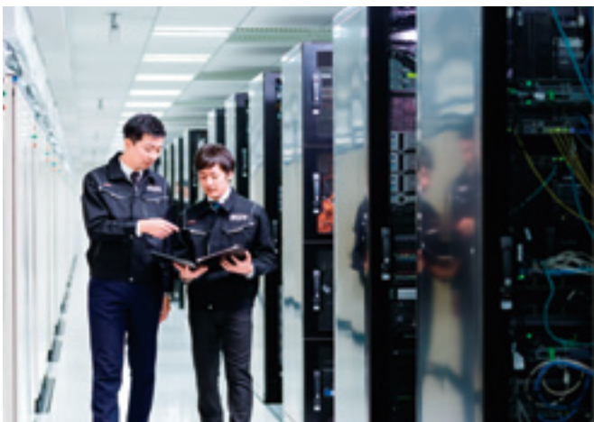
SECOM data center facility
