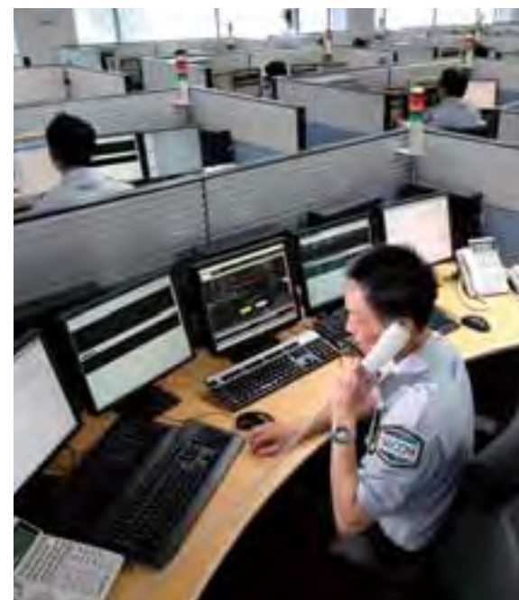
SECOM control center
