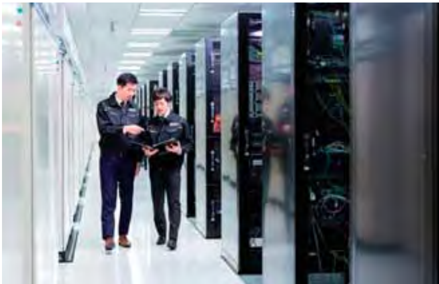
A SECOM data center facility
