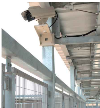
CCTV system installed in the center
