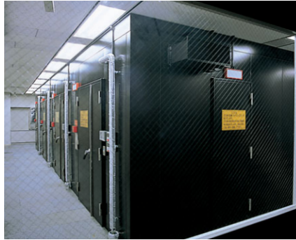
Secure Data Center storage area
