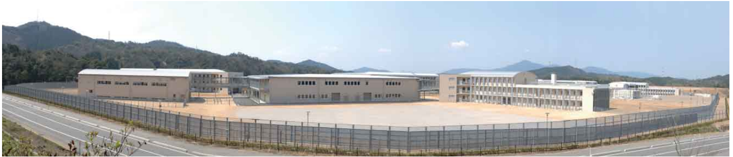
Mine Rehabilitation Program Center, Yamaguchi Prefecture
