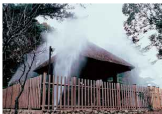
Fire extinguishing system installed to protect a cultural property
