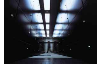
Secure Data Center
