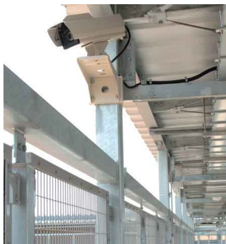
CCTV system installed in the center
