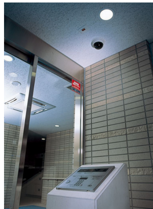
SECOM MS-3 condominium security system
