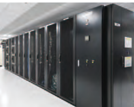
My Number information is stored at a Secure Data Center facility
