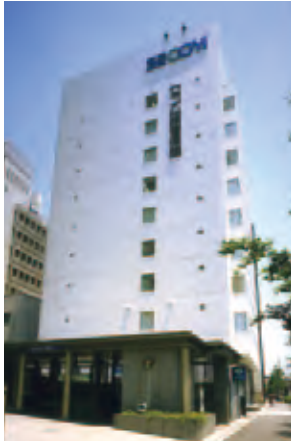
Headquarters of Secom General Insurance Co., Ltd.
