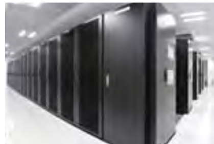
Secure Data Center
