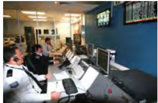
Control center (Secom Australia Pty. Ltd.)
