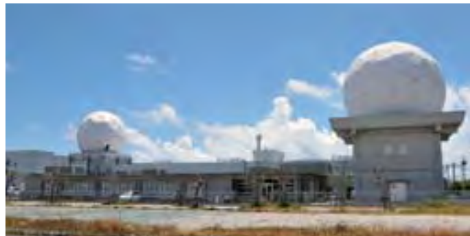
Satellite ground station (building with antenna) and geospatial information processing center (Okinawa)
