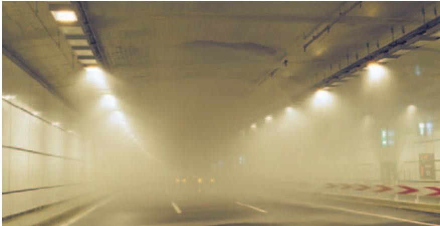
Water spray system installed in road tunnel
