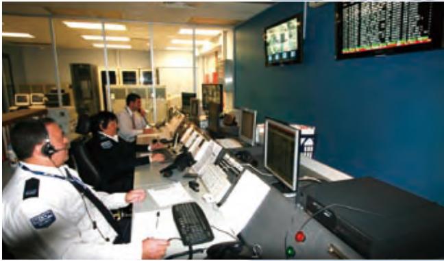
Control center (Secom Australia Pty. Ltd.)
