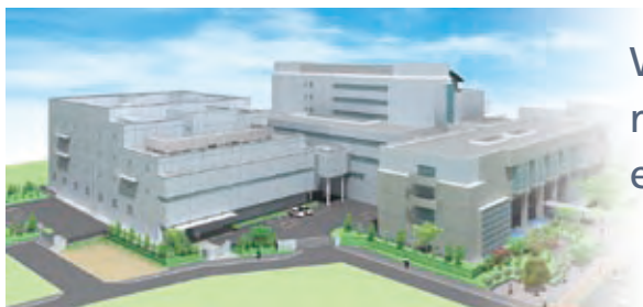
New Secure Data Center (left)
