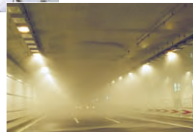
Water spray system installed in road tunnel
