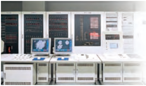
High-rise fire prevention center
