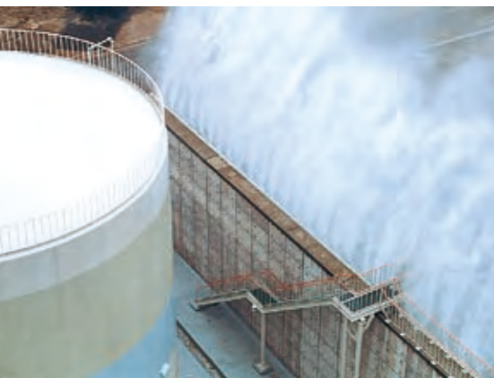
Water curtain system installed in tank yard
