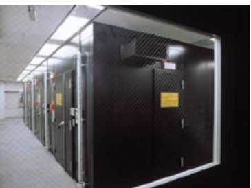
Secure Data Center
