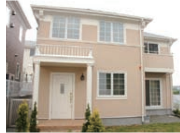
Built-for-sale house equipped with SECOM Home Security package as a standard feature
