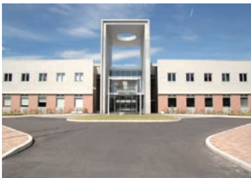
Exterior of the Kitsuregawa Rehabilitation Program Center, a PFI correctional facility
