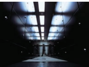
Secure Data Center
