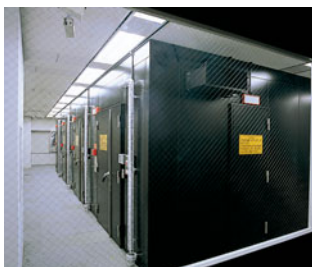
Secure Data Center
