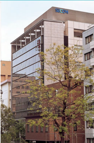
Yotsuya Medical Cube, which provides SECOM Health Care Club, a membership-based health management service, in an alliance with subsidiary Secom Medical System
