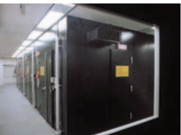
Secure Data Center
