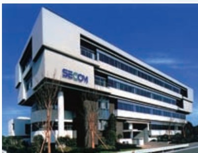
SECOM Development Center
