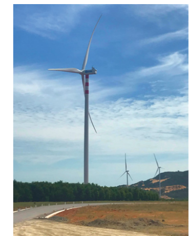
Wind power facility with Nittan fire alarm system in Vietnam's Ninh Thuận province (Nittan)
