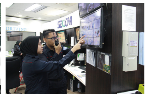
Control center (Secom (Malaysia) Sdn. Bhd.)
