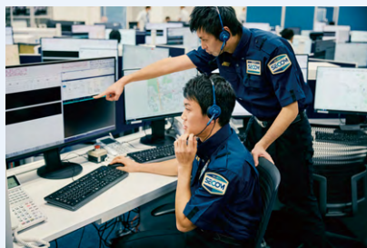
SECOM Control Center
