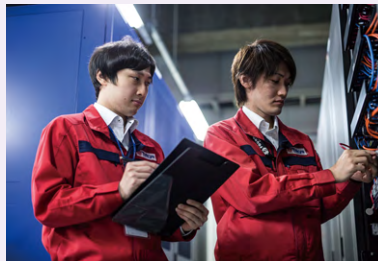
At Tokyo data center
