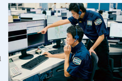
SECOM Control Center
