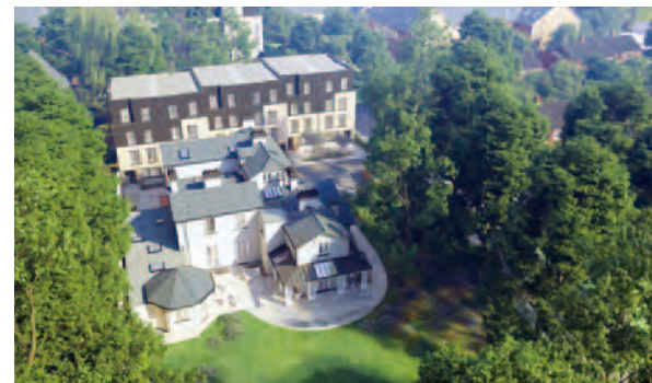
University student accommodation development in the United Kingdom that installed a Nittan fire detection system
