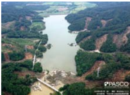
Aerial photograph of areas damaged in the 2018 Hokkaido Eastern Iburi Earthquake
