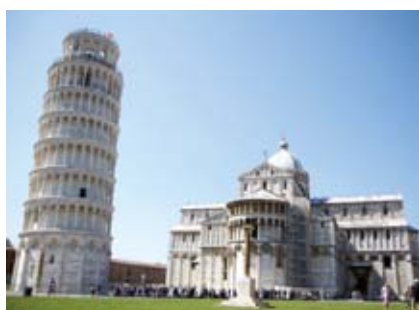
Fire protection systems installed at important facilities overseas (Nittan)
